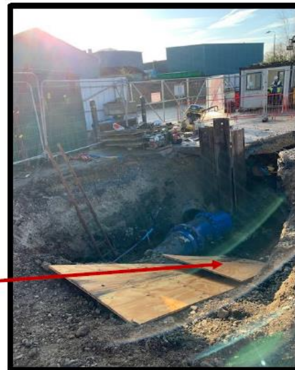
Open trench with rescue boards
